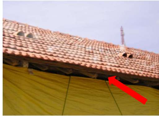
Pic 9: Curtain Hanging keeping Min Ventilation
