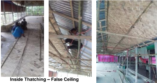
Inside Thatching – False Ceiling
