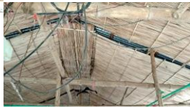
Inside Thatching – False Ceiling
