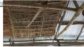
Inside Thatching – False Ceiling
