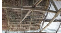
Inside Thatching – False Ceiling
