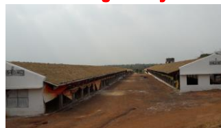
Outside - ASBESTOS Roof Thatching
